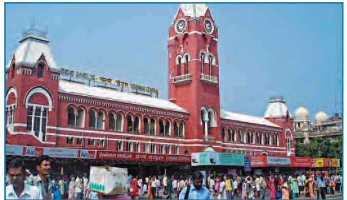
Chennai Central Railroad Station
